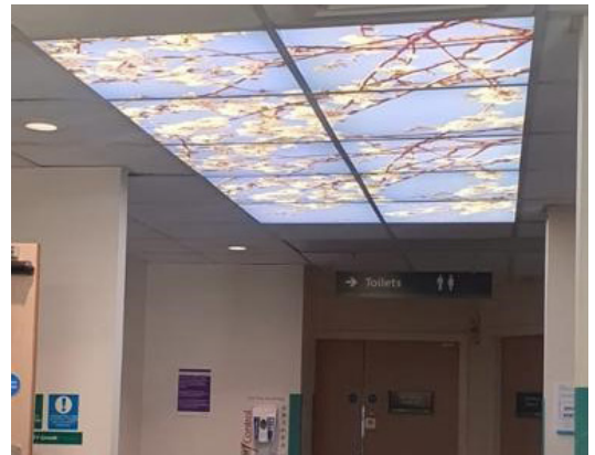
Skylight in the antenatal clinic
